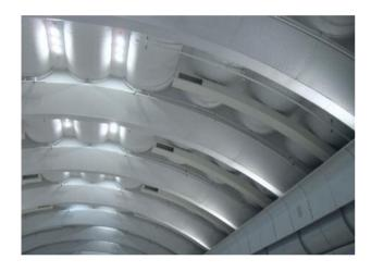
Kingspan Insulation commissioned a review by independent consultants, Rider Levett Bucknall, of the implications of reduced fan power on actual energy usage. Rider Levett Bucknall concluded that for a 328 ft / 100 m long run of ductwork, with cross–sectional internal dimensions of 24" x 24" / 600 x 600 mm and an air velocity of 1476 fpm / 7.5 m/s, ductwork fabricated from The *Kingspan* **Kool**Duct® System could save 10.5 MMBtu / 3100 kW·h per annum.
