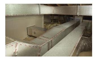
Traditionally, HVAC ductwork is constructed from galvanized sheet steel, which is installed first and then insulated separately as a second operation. The *Kingspan* **Kool**Duct® System however, is an advanced and innovative pre–insulated rectangular HVAC ductwork system, which is installed in a single–fix.
